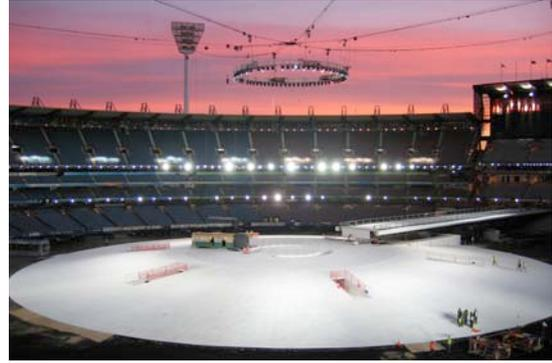
ARENA: 7 metre diameter central lift with 12 tonne capacity
