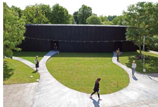
Groundworks: We provided curved paths and festoon lighting
