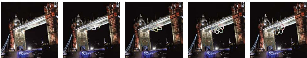
AUTOMATED: The rings took around three minutes to lower, lifting when required to allow the bascules to open and let the river traffic through.
